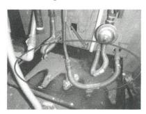
The condensate drain line is not plumbed to the exterior drain.
