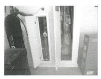
The interior garage wall enclosures are a breach in the required fire separation of the interior garage walls. -Not less than  $^{1}$ /<sub>2</sub>-inch gypsum board or equivalent applied to the garage side of structural members supporting the floor/ceiling assemblies or garage ceiling. Structural members include, but are not limited to: walls, columns, beams, girders, and trusses.
