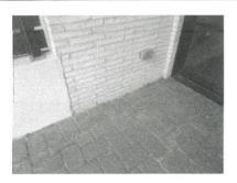
Grade is in contact with exterior cladding or lacks 4" of clearance to masonry walls or 6" of clearance to all other siding materials as required by [IRC R404.1.6]. This condition will permit water intrusion into the wall assembly, water damage to structural elements, and is considered to be a conducive condition for termite infestation.
