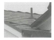
Plastic roofing tiles are not installed flush to the roof surface and may be subject to wind lift and storm damage.
